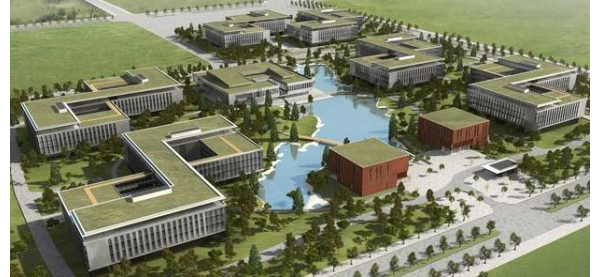
Airscape of HUAWEI, located in Hangzhou, China
